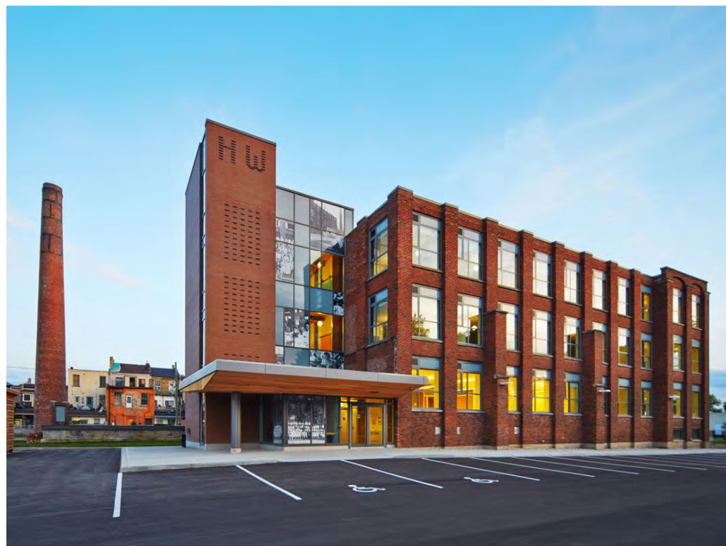
Queen's Park Pick for Oxford County: Harvey Woods Lofts, an adaptive reuse affordable housing project by Invisij Architects.
